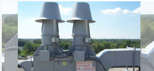
Roof Top Exhaust unit
