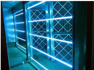
Ultraviolet Light (UV) located in Air Handler
