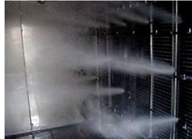
Humidification (in air handler)
