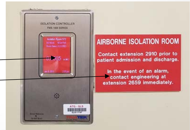
Air pressure monitor/alarm with signage
